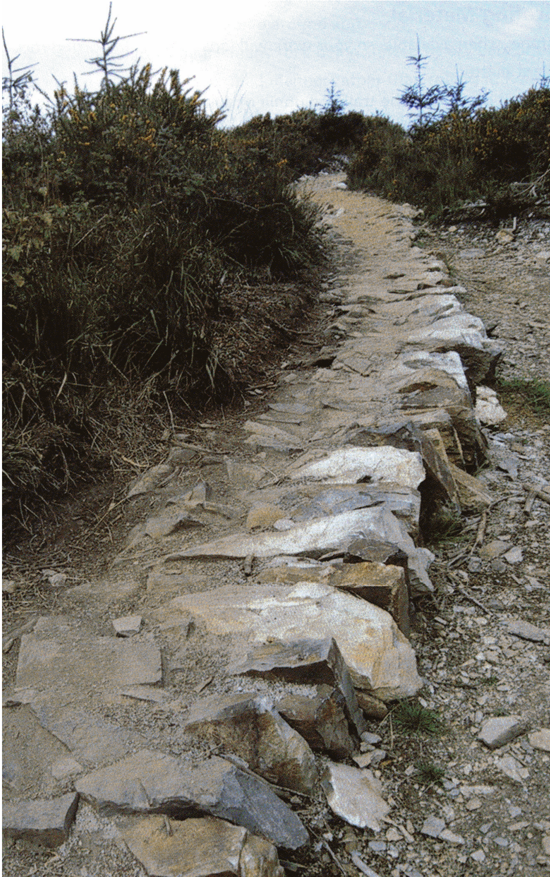
An example of a finished stone pitched surface.
