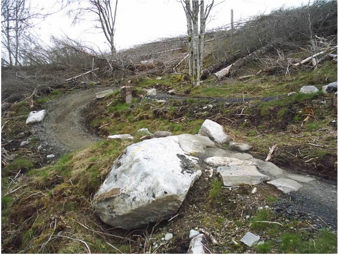
An example of where natural features have been incorporated into the trail construction, this principle should be adopted on the Carron Valley project where appropriate.
