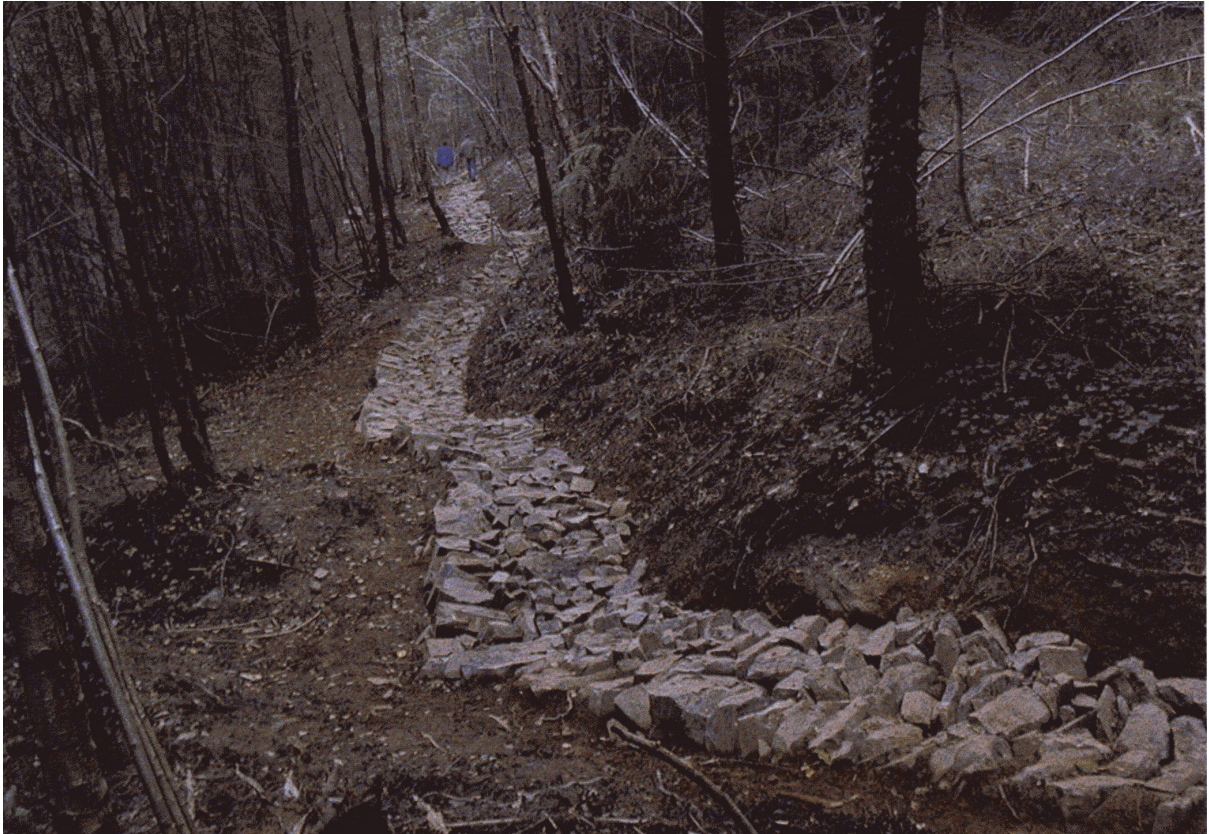
A typical stone fill example prior to the surface coat being applied i.e. the finer material.
